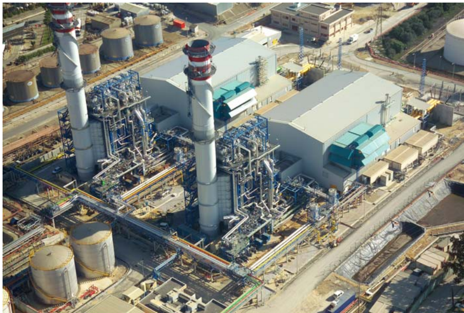
Aerial Photograph of the NGS Power Station showing the two CCGT plants.
